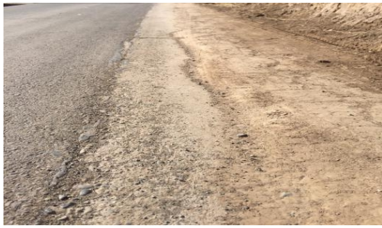
尖山村人饮管网地表恢复
