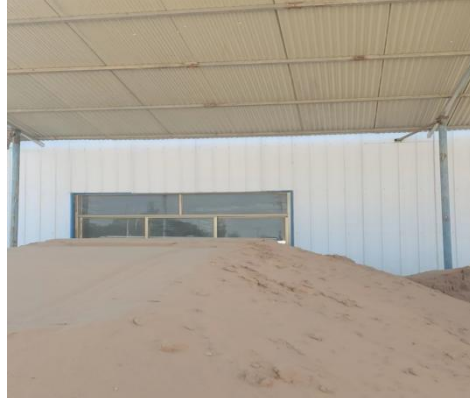
半封闭原料棚
