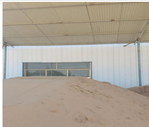
半封闭原料棚
